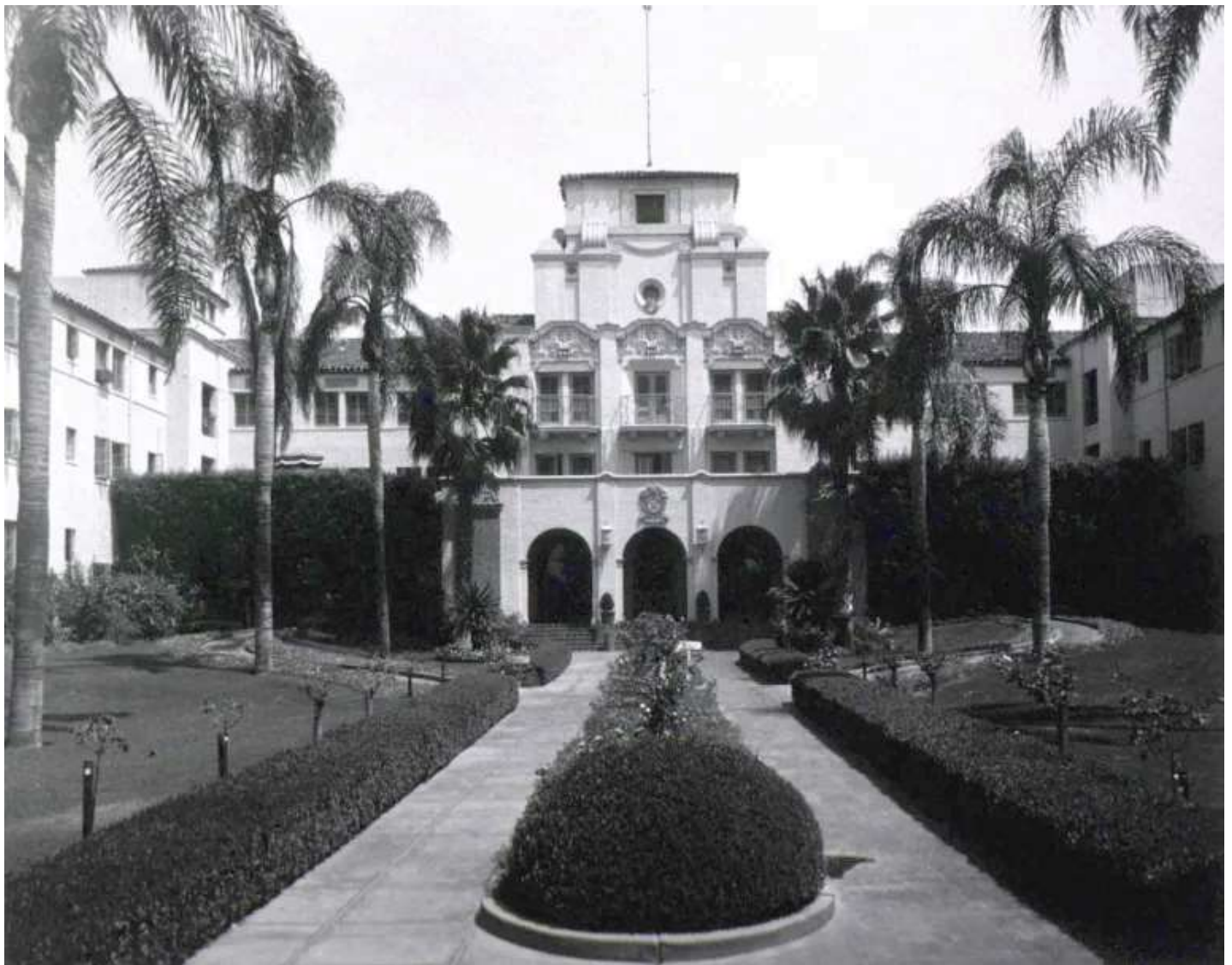
The Entrance to the Norconian "Clubhouse," 1951.
